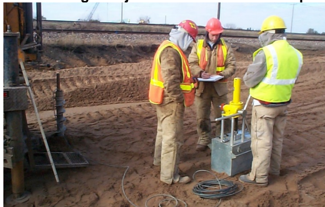
Figure 3-8 Pressuremeter testing being performed to assess soil conditions for the Glen Road Interchange Project on US10/US61 in Newport, MN
