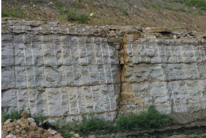
Figure 8-2 Rock face blasted with controlled blasting
