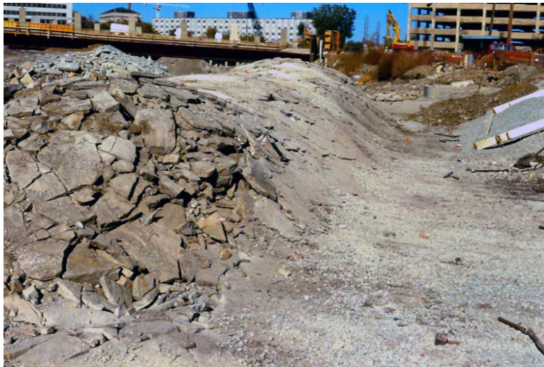
Figure 8-1: Production blasting showing movement (bulking up) of the rock
