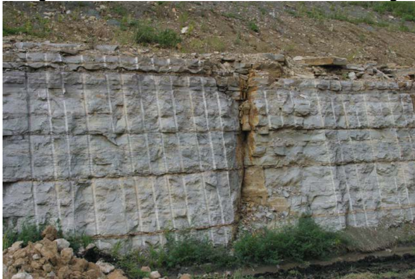
Figure 8-2 Rock face blasted with controlled blasting
