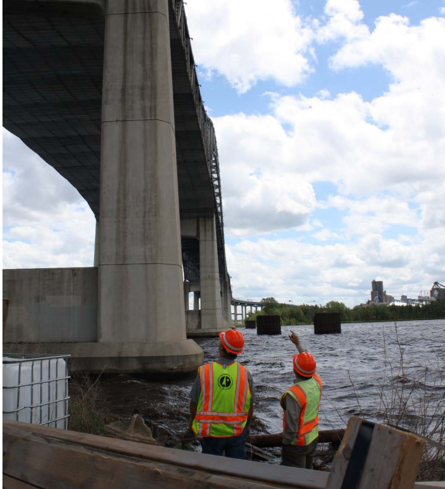
Figure 16: Workers examining the Blatnik Bridge
