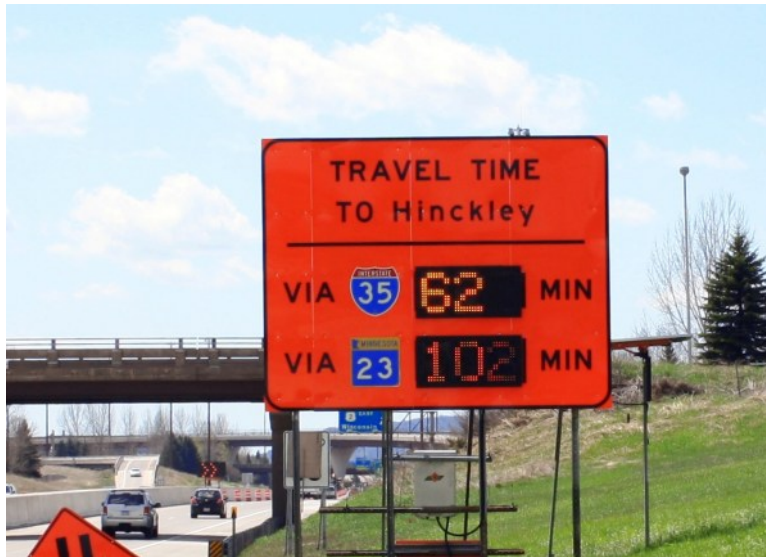
Figure 27: Travel time sign for construction-related congestion
